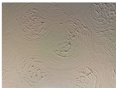
Older decorative ceilings, like this one, often contain small amounts of white asbestos.
