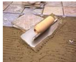
Picture of asbestos floor tiles and asbestos flooring paste.
