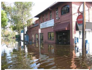
Flood damaged shopping center
